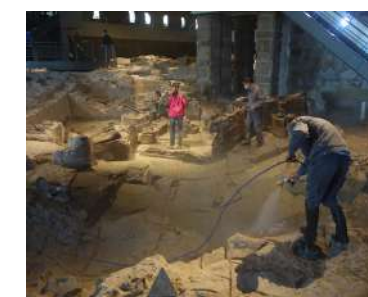
New type protection of nano-silica spraying and coating on site
